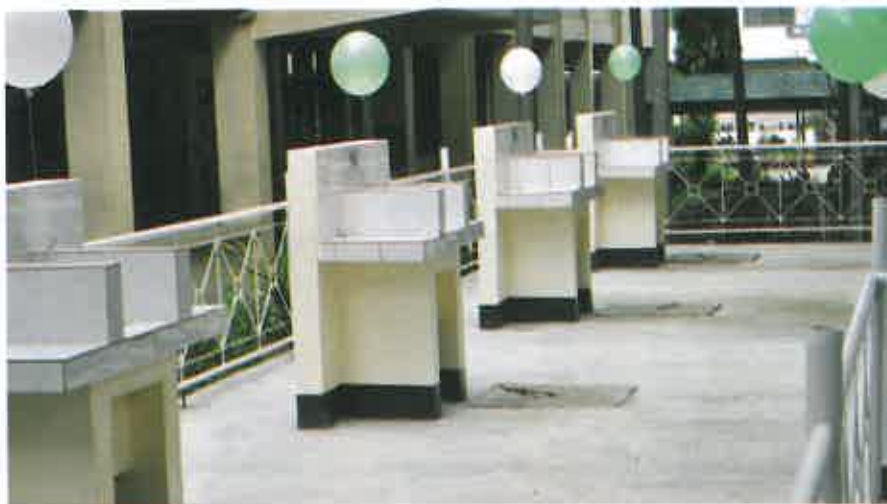
Figure 9. RAINWATER HARVESTING UNIT
